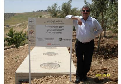
In addition to classic SBR systems, a new generation of load-controlled SBR (Puroo) has been installed at house level. The system works without electric pumps and valves. Since the operation is carried out with compressed air, the energy requirement of the technology is very low (30 kWh per inhabitant per year).
